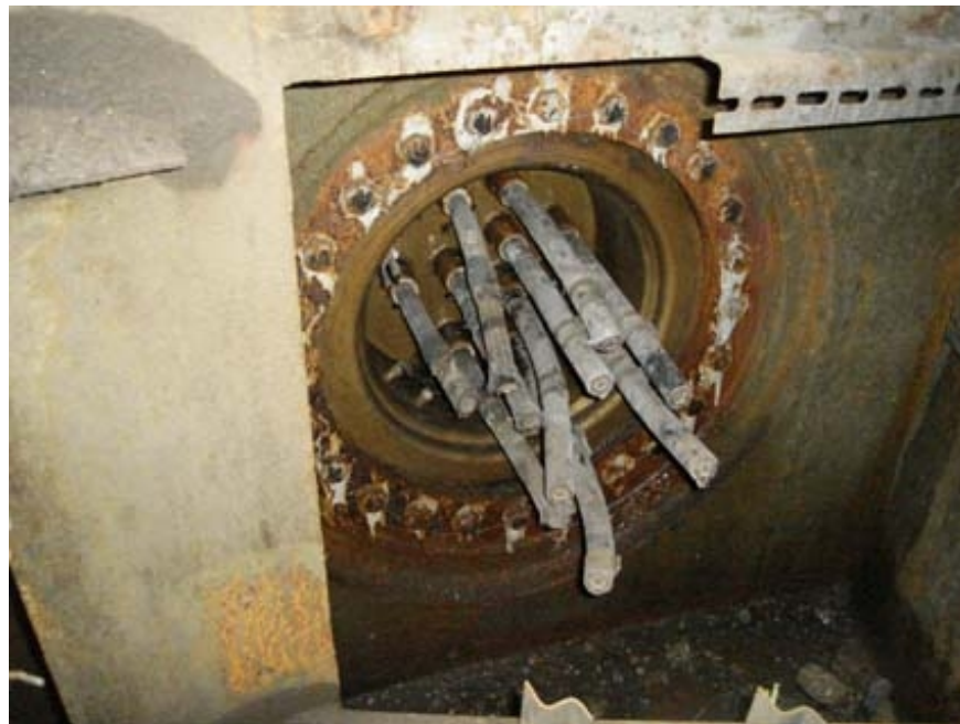
Figure 8 Signal cables in the underground gallery to the antenna "Bruschatka"
