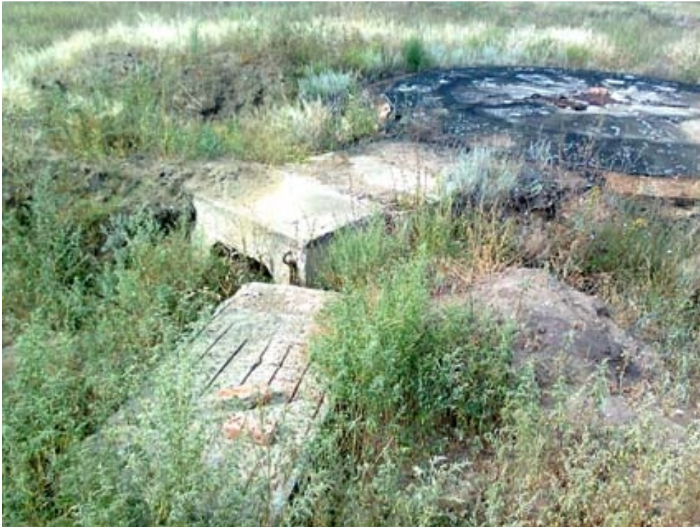
Figure 7 Another view of the destroyed Antenna "Bruschatka"
