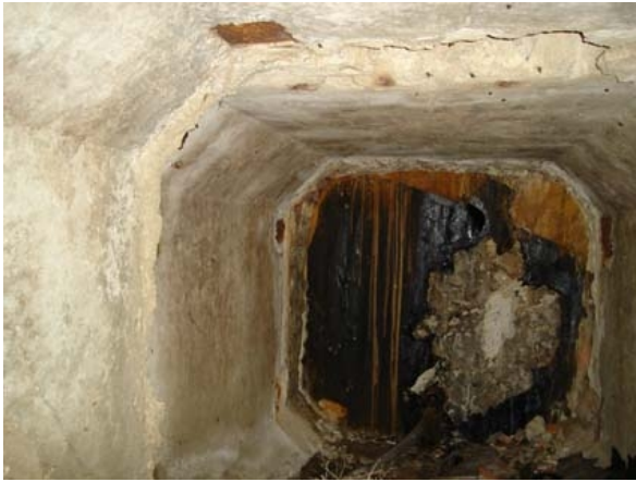
Figure 4 Underground gallery to the antenna with some strange metallic lustre mastic
