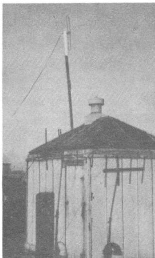
THE ANTENNAS AT WLOOP. TOP, THE "TROMBONE" (FOLDED DIPOLE). AT THE LOWER CENTER, THE 220 MCS. 4-ELEMENT YAGI. SEE PAGE 6.
